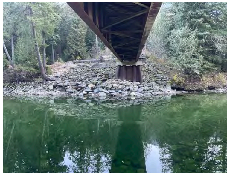
Right face of main span pier
