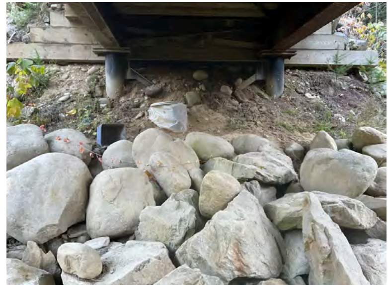
Left Bank Abutment when facing downstream
