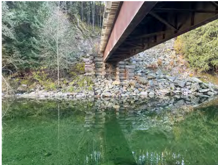
Right Bank Abutment when facing downstream
