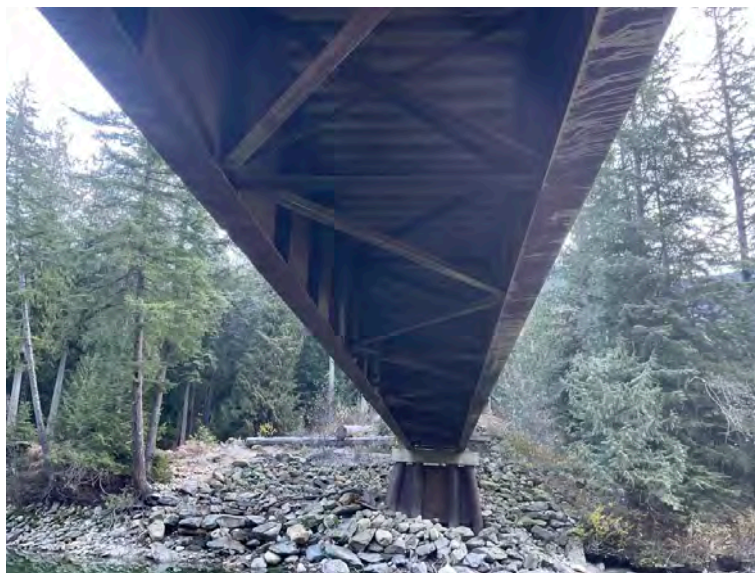
Main span superstructure
